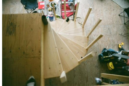
Figure 10 - Spiral staircase made from downed tree and installed in the cabin.
