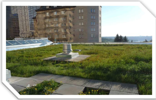
Figure 3: The William Engineering Green Roof
